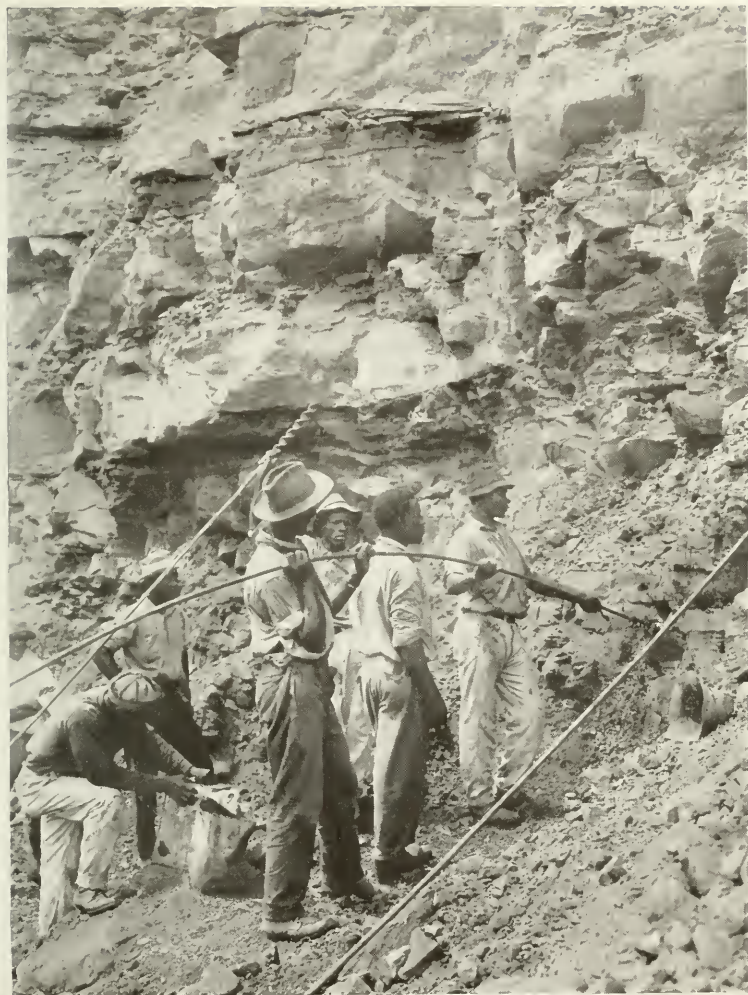
HAND DRILL GANG BORING HOLES FOR DYNAMITE TO BLAST MOVING FACE OF A "SLIDE" IN THE CULEBRA CUT, FEBRUARY, 1912.
